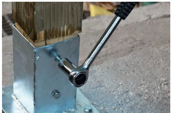
STEP6. Using a wrench key to drive screws.
