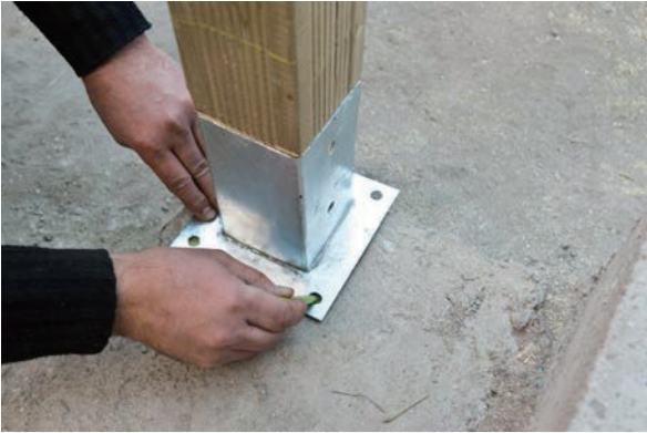
STEP1. Marking where to install post anchors.
