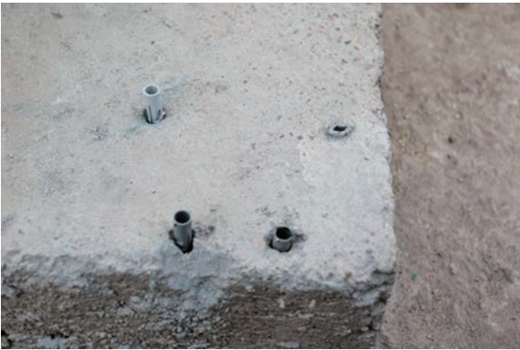
STEP3. Installing dowels in concrete.
