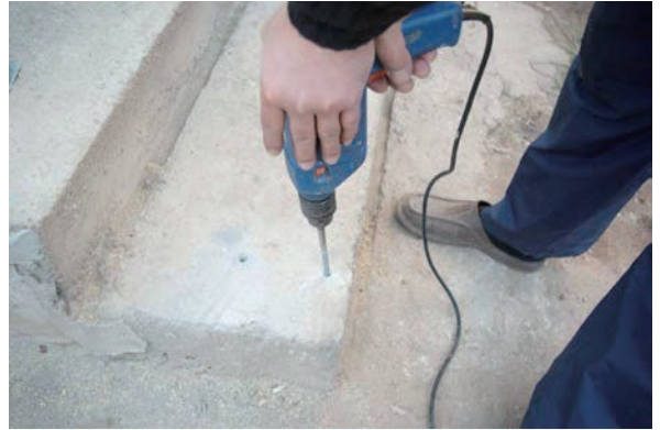
STEP2. Drilling holes to anchor the post.
