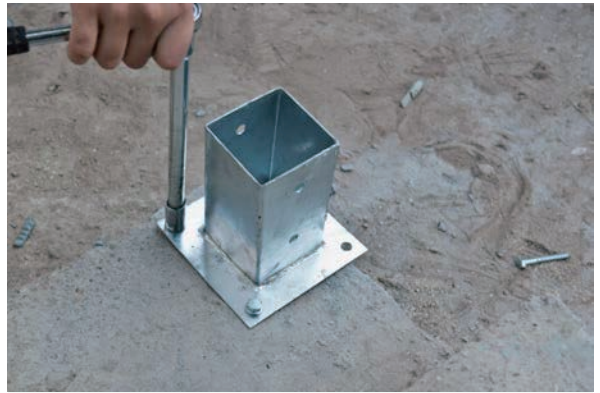
STEP4. Installing post anchor.
